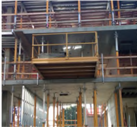
"Cantilever Cargo Platform" allows for safe movement of material using passive Fall Protection
