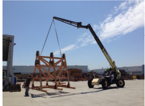
"Wall Panel Storage Rack" to facilitate the storage and safe access of wall forms
