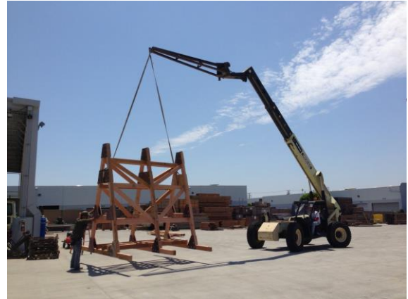
"Wall Panel Storage Rack" to facilitate the storage and safe access of wall forms
